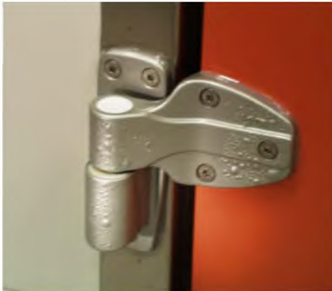
Paint blistering of surfaces and floors
