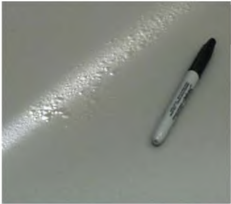
Paint blistering of surfaces and floors
