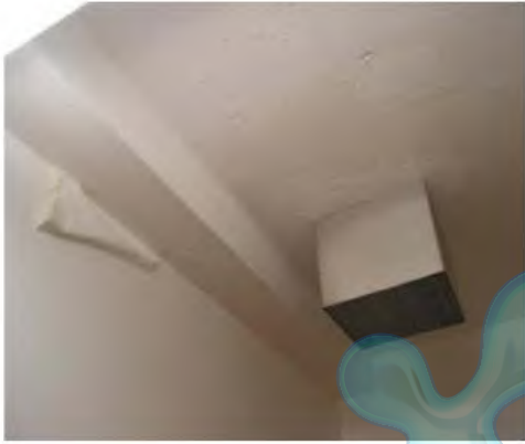
Paint blistering of surfaces and floors
